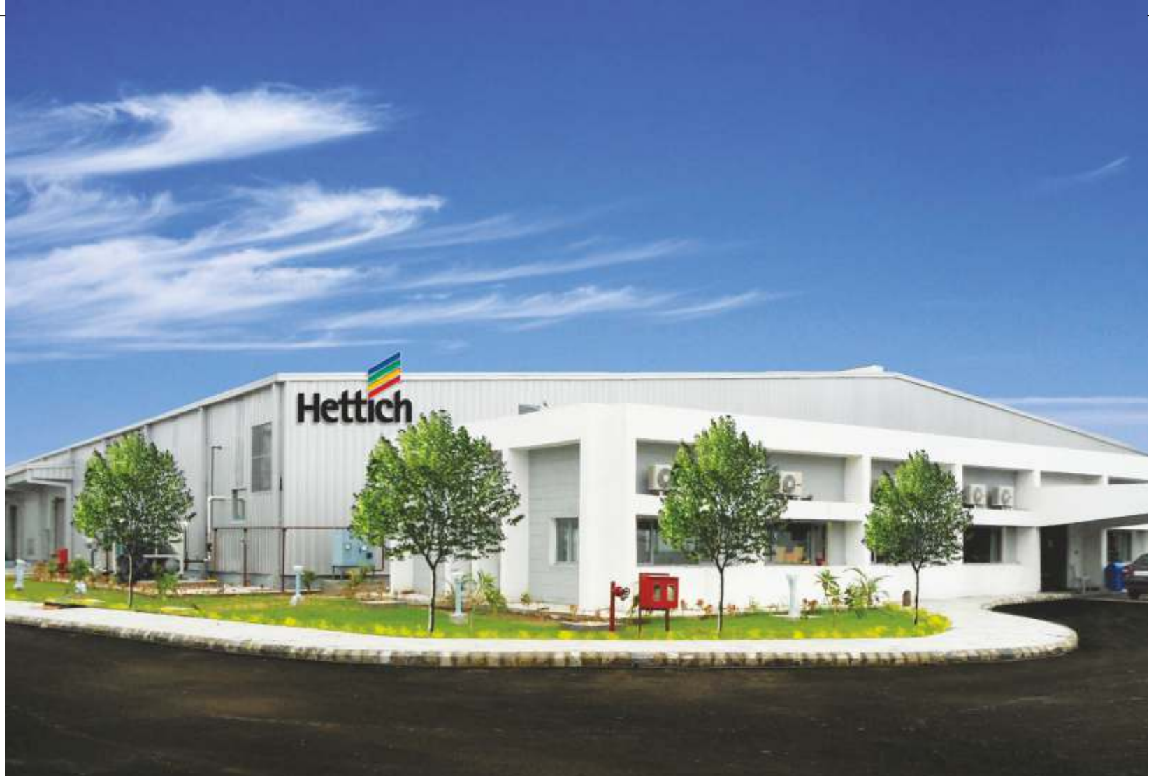
Hettich Manufacturing Unit at Vadodara, India
